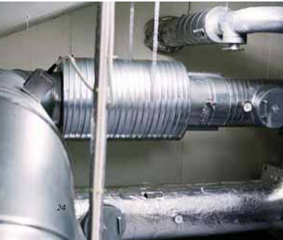
Example of an insulated duct (bottom duct). The two ducts above have silencers
