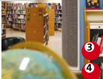
Floor-installed diffuser with exhaust air diffuser in ceiling.
