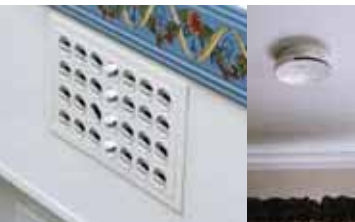
Ceiling and wall-installed diffusers.
